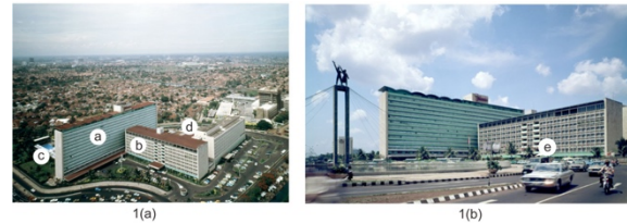
Figure 1(A-B) The top view of the Ramayana Wing building (a) and Ganesha Wing (b) form T-shaped after being completed around 1962 (A). Behind the Ramayana Wing building is the Ramayana Terrace (c) and Bali Room behind the Ganesha Wing (d). Photo (B) shows the location of the emergency exit of the Bali Room Foyer (e) which becomes the site location of Margasatwa dan Puspita Indonesia paintings after the renovation until now. Photo: Hotel Indonesia Kempinski.
