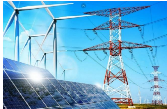
Figure 2 Windmills and solar panels.
