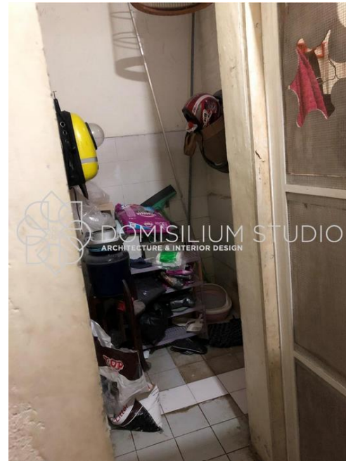
Picture 2: Interior Existing in front of Bathroom Area (Source: Domisilium Studio Archives)
