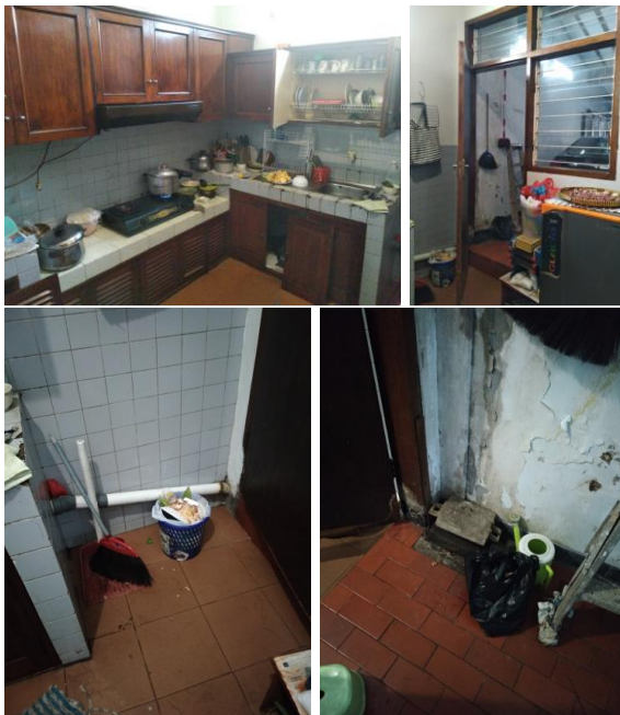
Figure 5: Existing Kitchen Condition (by Author Team, 2019)
