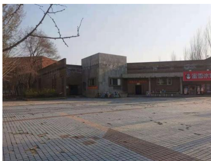
Figure 1 Square in front of the boiling water room
