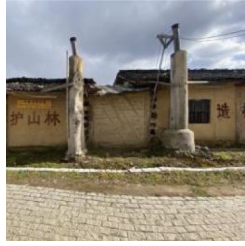
Fig. 7. Iron-Wood Mixed Chimney
