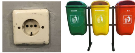
Fig. 4. The condition of the equipment in Computer Drawing Laboratory of SMK Negeri 2 Salatiga.
