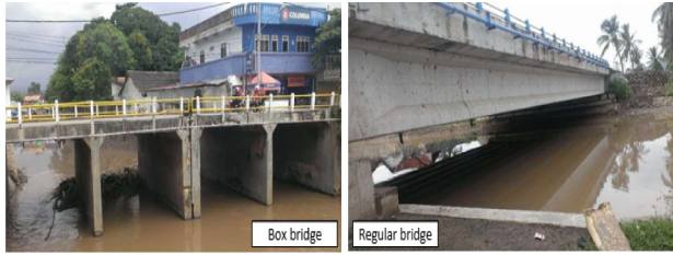
Fig. 9. Comparison of box bridge and regular bridge; a bridge consist of boxes, their capacity transferring flow during flood will be reduced by the trapped floating objects.
