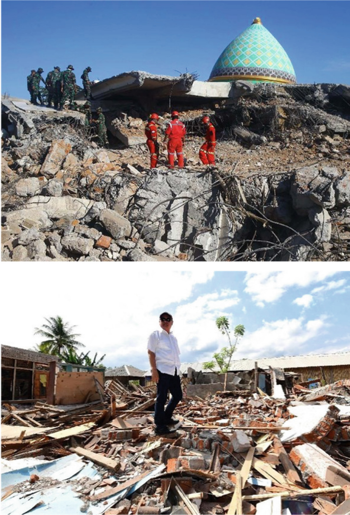
Fig. 2. The impact of Lombok Earthquake on 2018 which damaged most of the resident's houses in North Lombok [15].
