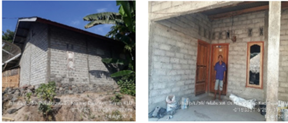
Fig. 13. Condition of House Building with adequate quality concrete material
