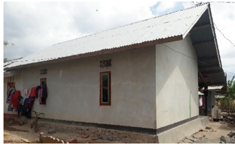
Fig. 14. The type of gable roof used by the majority of the people of North Lombok
