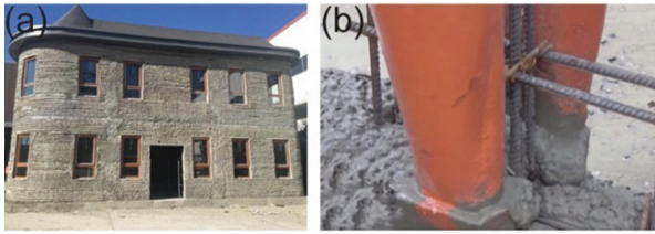
Fig. 2. (A) The two-story villa 3D printed by Huashang Tengda company; and (B) the novel nozzle of the giant 3D printer (Sanjayan, 2019)
