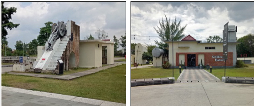
Fig. 4. Condition of De Tjolomadoe Complex in 2021 (Doc. Research Team, 2021)
