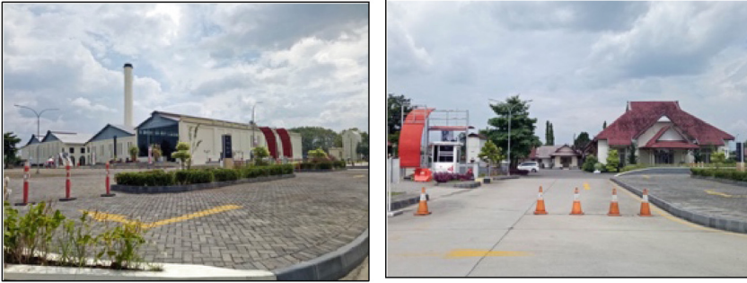
Fig. 3. Condition of De Tjolomadoe Complex in 2021 (Doc. Research Team, 2021)
