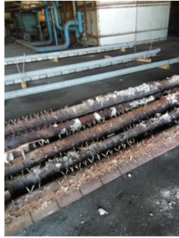
Fig. 12. Skid Rail Pipe
