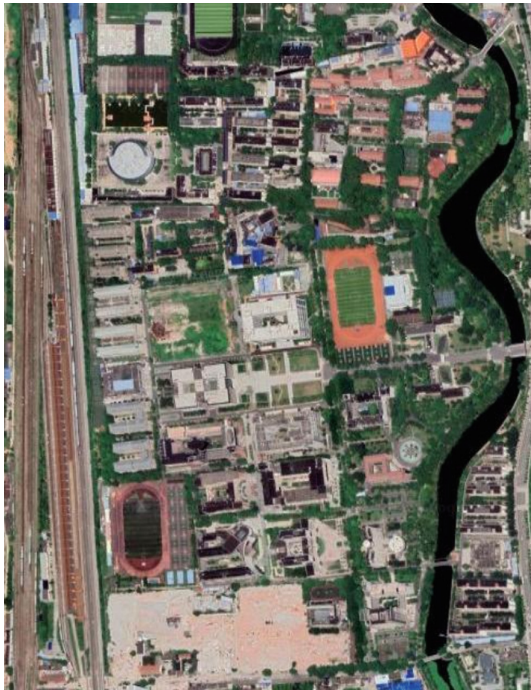
Fig. 1. Campus satellite image (Image source: intercepted by Google Maps)
