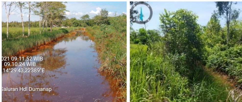
Figure 4 The existing condition of Handil Dumanap, which is still functioning (left), and Handil Gardu, which has been overgrown with vegetation (right)
