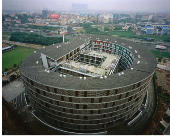
Fig. 9. The exterior view image and middle courtyard for collective use of Urban Tulou. [ https://architectureindevelopment.org/project/346 ]
