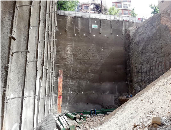
Fig. 3. The support system used for stabilization
