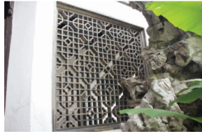
Grinding Brick Latticed Window
