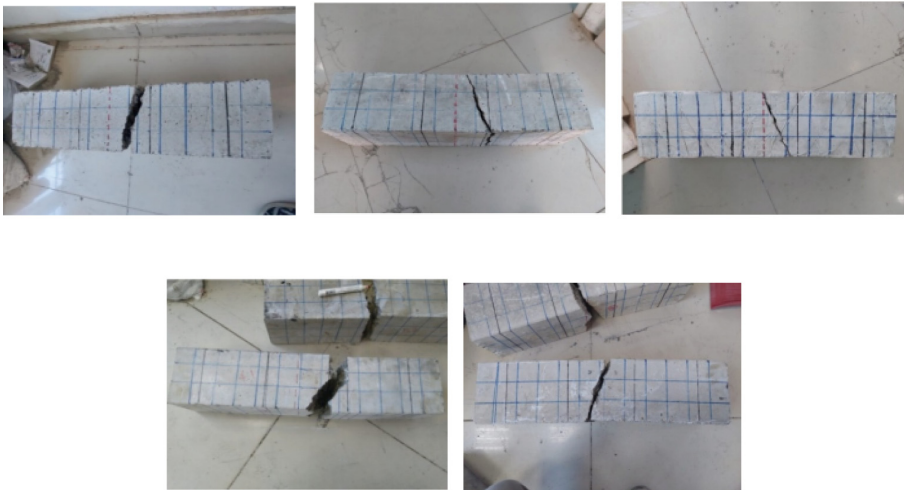
Fig. 4. Example of crack pattern of beam specimens
