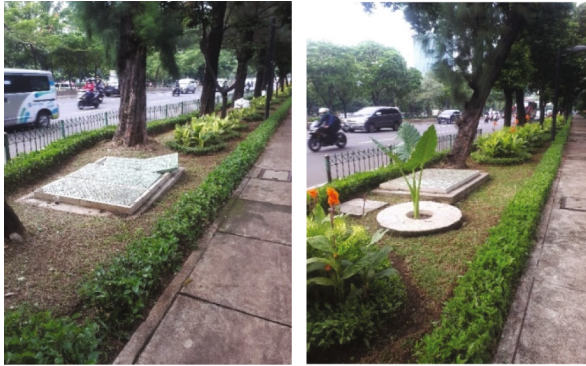
Fig. 3. Existing Condition of Pedestrian Paths.
