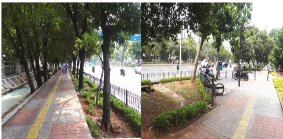
Fig. 2. Existing Condition of Pedestrian Paths.
