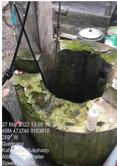
Fig. 4. Dug well condition in Gumpang Village
