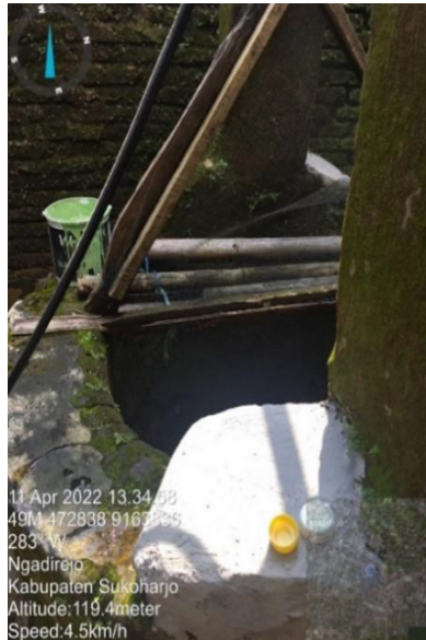
Fig. 3. Dug well condition in Ngadirejo Village
