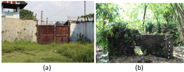
Fig. 3. SCS facilities at Sindanglaut factory Fasilitas Perkeretaapian SCS di Sindanglaut: (a) Gateway for lorry; (b) Abutment structure for railway bridge (Source: Balai Arkeologi Jawa Barat, 2018)
