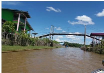
Fig. 13. The elevation of the bridge is made high on the channel that is used as a water transport channel
