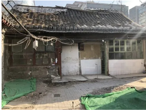
Fig. 5. Ningqiang Guild Hall(Exterior)
