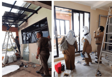
Fig. 6. Water panel repair, building repair and underground rooms.
