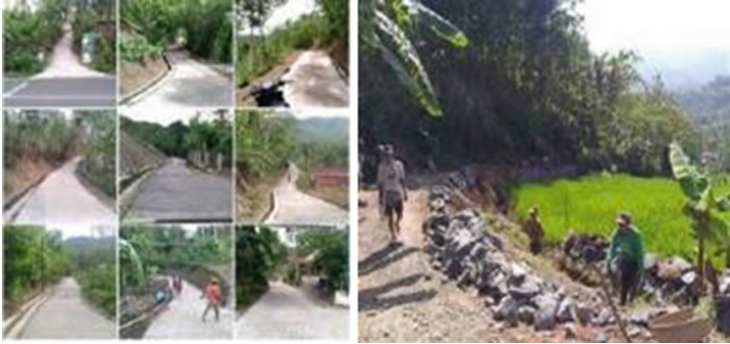
Fig. 3. Road conditions in Karanggayam district.
