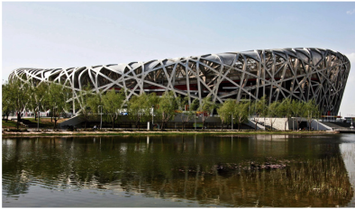
(c) Beijing National Stadium
