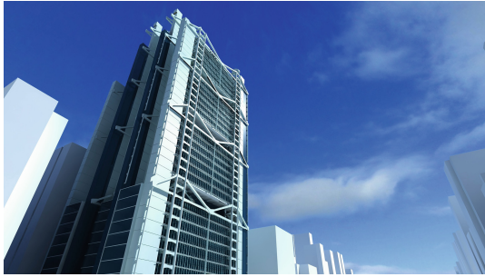
Fig. 3. HSBC Bank Building
