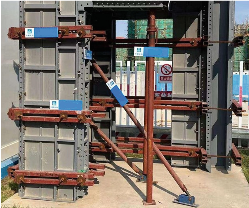
Fig. 1. Tie-rod cantilever scaffolds
