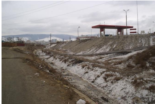
Fig. 6. Petrol station 'Petrovis' company.
