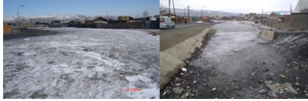
Fig. 3. Dam covered with ice and filled with household waste.
