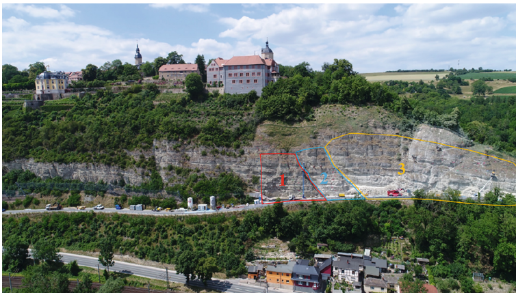
Fig. 13. Division of the wall into three structural complexes
