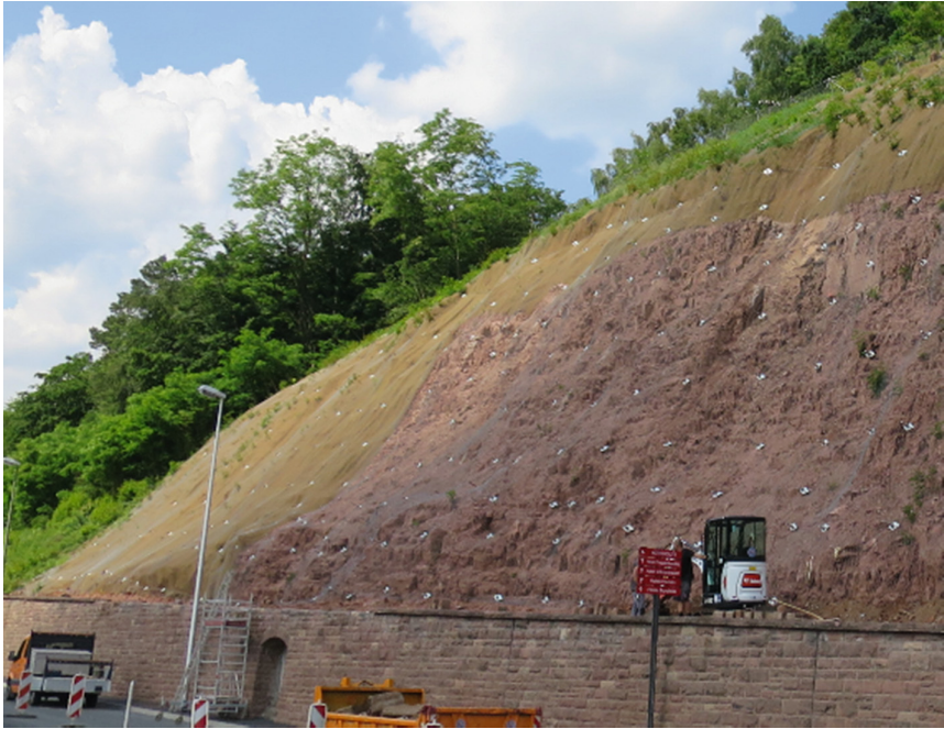
Fig. 10. Construction after completion with erosion protection mats applied in certain areas.
