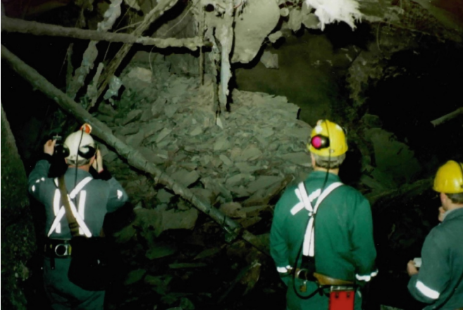
Fig. 7: Back collapse resulting from an \sim M_L 3.0 mine induced seismic event
