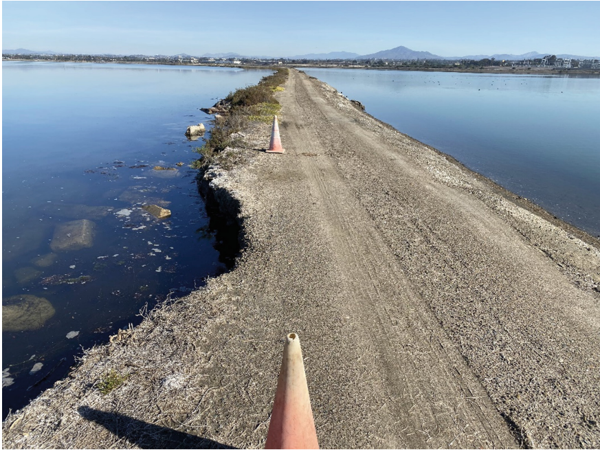
Fig. 3. Site photograph of existing Berm 15
