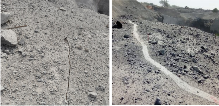
Fig. 1. Development of tension crack and before monitoring crack was sealed and glass strips were put
