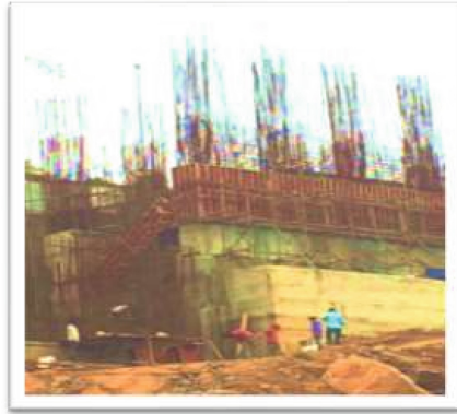
Fig. 5. Progress of Construction of Retaining Wall
