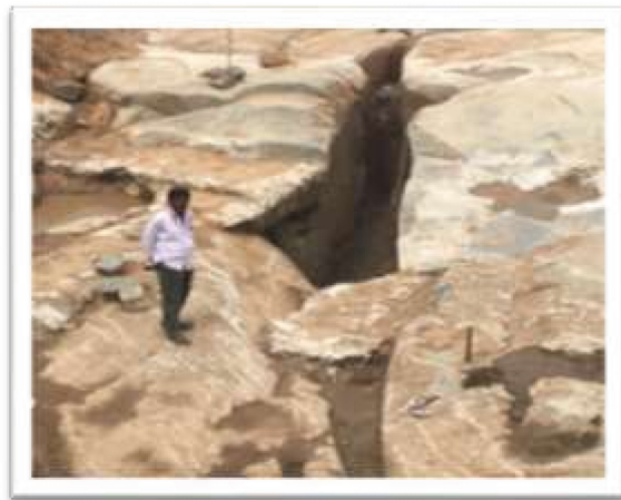
Fig. 6. Foundation Area for the Main Gateway
