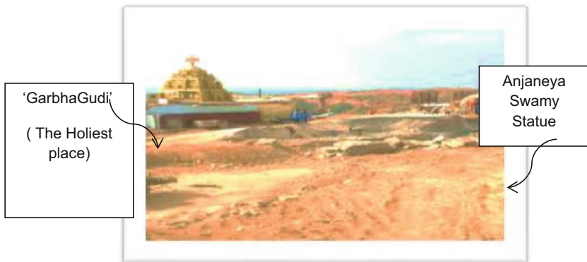
Fig. 1. Dismantling the Temple
