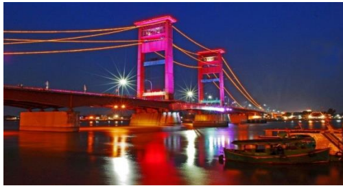
Fig 2. Ampera Bridge. Source: Palembang.go.id (2023).
