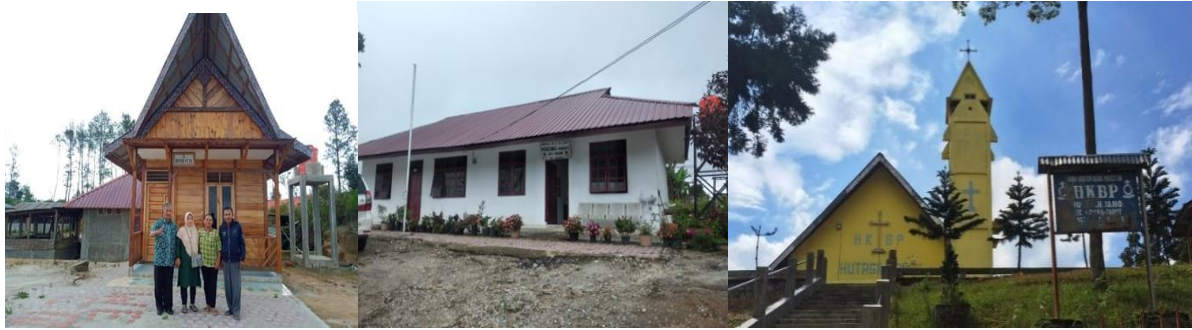
Fig. 6. Facilities in Huta Ginjang village (Lodging, Health Center, HKBP Church). Source: Researcher (2022).
