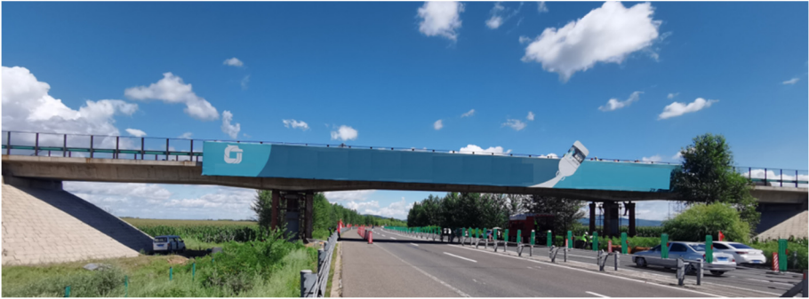
Fig. 1. The real picture of the single-column pier bridge
