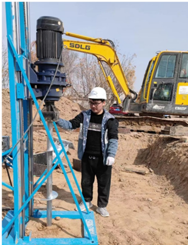
Fig. 4. Professional piling. equipment.
