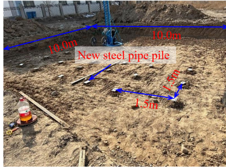
Fig. 1. On-site excavation and test pile layout.
