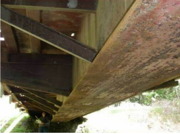
Fig. 1. Corrosion diagram of steel structure
