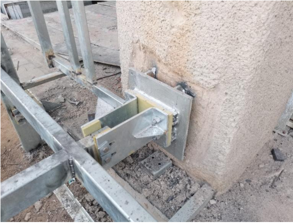
Fig. 6. Construction Drawing of Moisture-proof and Heat-insulating Gaskets
