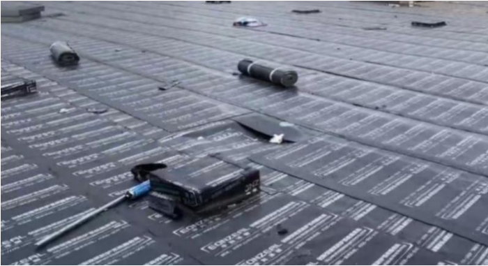
Fig. 4. Paving Diagram of the Waterproof Membrane
