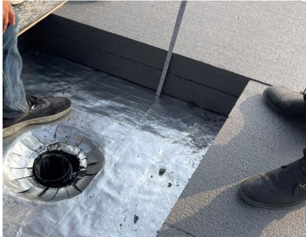
Fig. 2. Paving Diagram of the Staggered Assembling of Graphite Polystyrene Board
