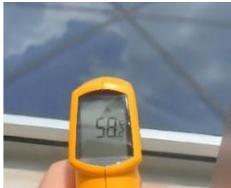
(b) The temperature of the outer wall surface of the skylight at the top of the atrium.
