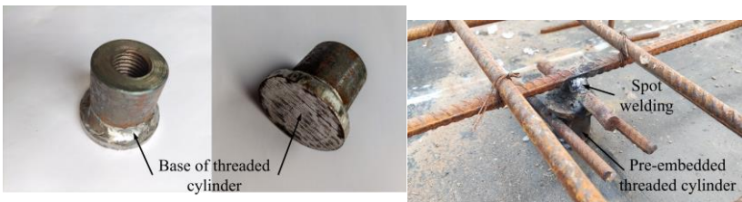
(a) Pre-embedded threaded cylinder (b) Fixing method of pre-embedded threaded cylinder
