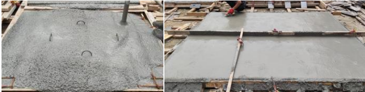
(a) Vibration of concrete
