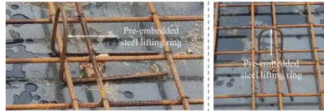
Fig. 12. Pre-embedded reinforcement rings
