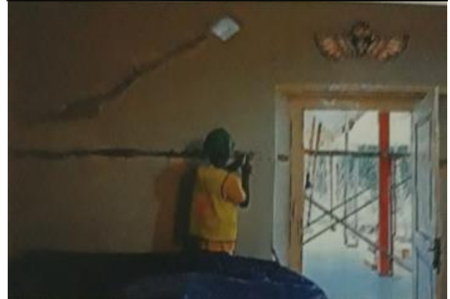
Fig 4. The Wall Breaking Work of the Parangkarsa Building
