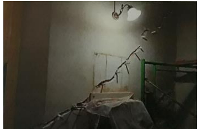
Fig 5. Pipework for Sikagrout Injection
