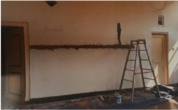
Fig 6. Final results of grouting work
