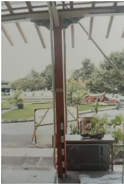
Fig 2. Replacement of saka wood (columns) in the Gandhok Kilen Building
