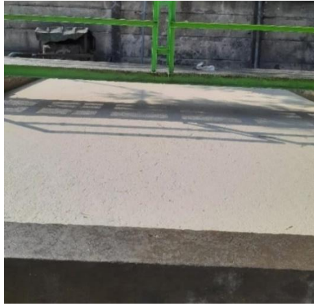
Fig. 6. Sedimentation Basin Construction
