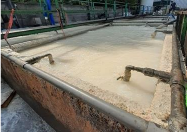
Fig. 5. Aeration Basin Construction
