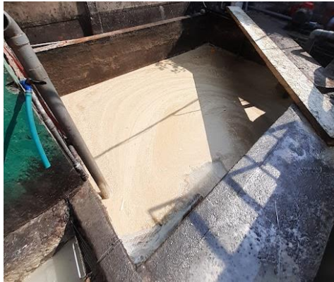
Fig. 2. Equalization Basin Construction
