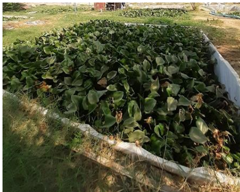
Fig. 7. Constructed Wetland Construction
