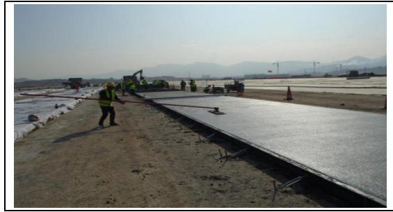
Fig. 11. Illustration of One Pass with Large Iron Trowel in Texture Dragging
