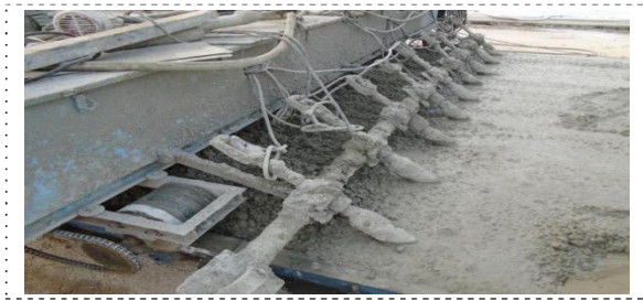
Fig. 6. Detailed Illustration of Concrete Compaction (Vibration) Construction
