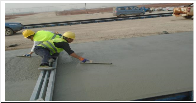
Fig. 10. Wood Troweling Operation
