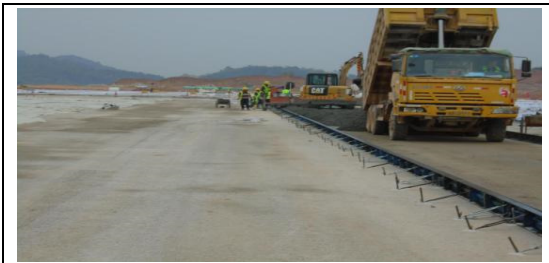
Fig. 4. Concrete Unloading and Paving
