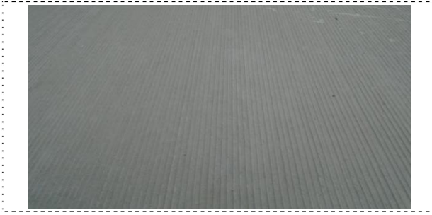
Fig. 14. Finished Texture Depth Effect
