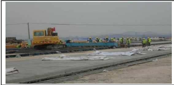
Fig. 3. Concrete Paving Construction
