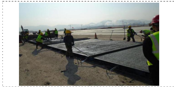
Fig. 8. Roller Troweling Operation
