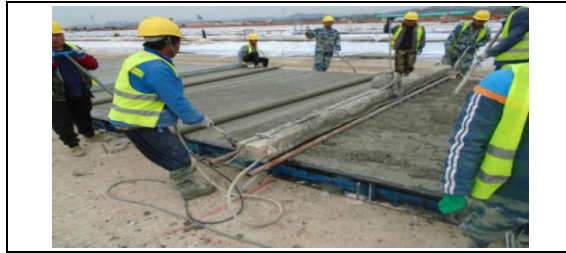
Fig. 7. Vibrating Beam Surface Leveling and Slurry Work
