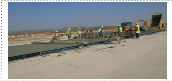
Fig. 5. Concrete Compaction (Vibration) Construction
