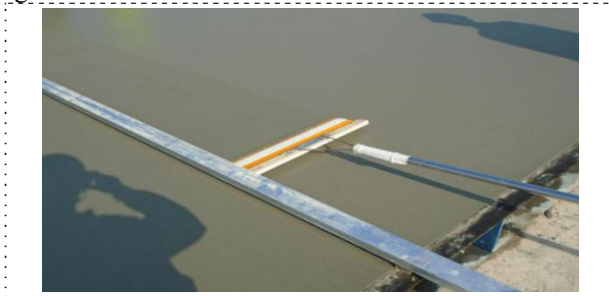
Fig. 13. Texture Dragging Process Illustration
