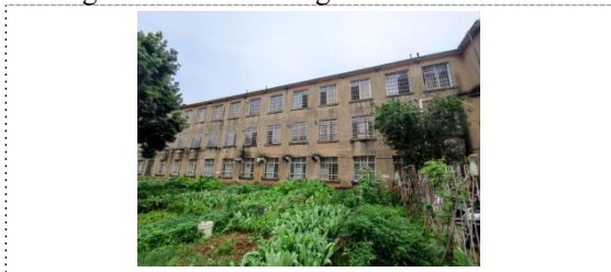
Fig. 1. Current situation of old buildings
