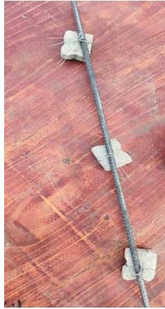
Fig. 8. Modularized Concrete Spacer Blocks (1)
