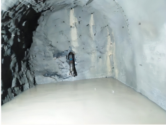
Fig. 6. Accurate penetration of the field guide hole
