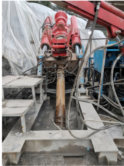
Fig. 5. Backward well drilling site construction
