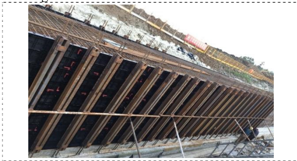
Fig. 9. Steel-plastic composite template assembly effect.
