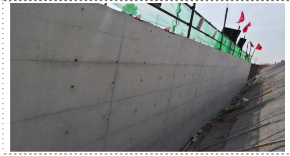
Fig. 10. Appearance of concrete after mold removal.
