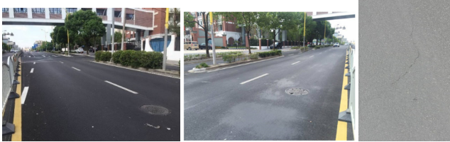
Fig. 7. Pavement condition after one month (from left to right: LFT; GT; RL).
