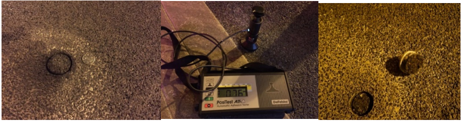
Fig. 10. Pull-off test in the field.
